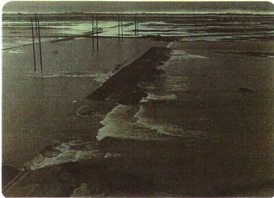
PHOTO 42 WEST CHANNEL SAGAVANIRKTOK RIVER Looking at gravel roadway sections (crossing overflow channels from the West Channel) overtopped by the 1981 breakup flows. Culverts in between the overflow sections have inadequate capacity. 65-7-0
