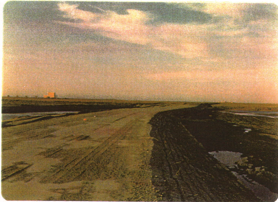
PHOTO 44 KUPARUK RIVER View of designed overflows. "Armorflex" articulated concrete blocks (12" X 12") on upstream and downstream faces of embankment and a concrete driving surface. 65-14-10 July 1982
