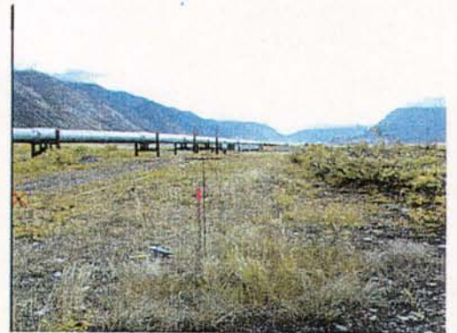
TAPS - Pump Station 4 area
