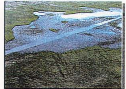
Ponding over Nuiqsut gas pipeline.
