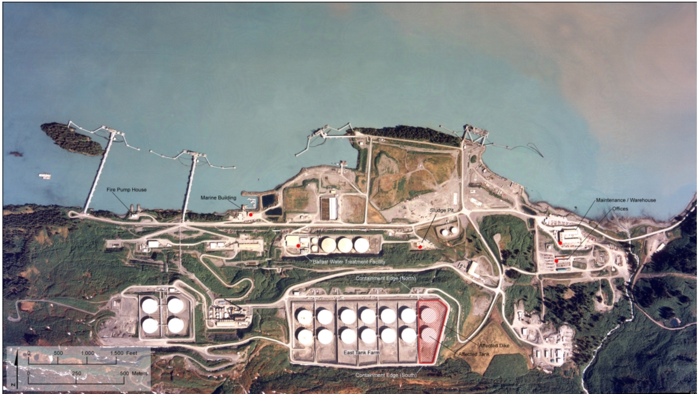
FIGURE 4.4-2 East Tank Farm Facilities Potentially Affected in the Valdez Marine Terminal Fire Scenario
