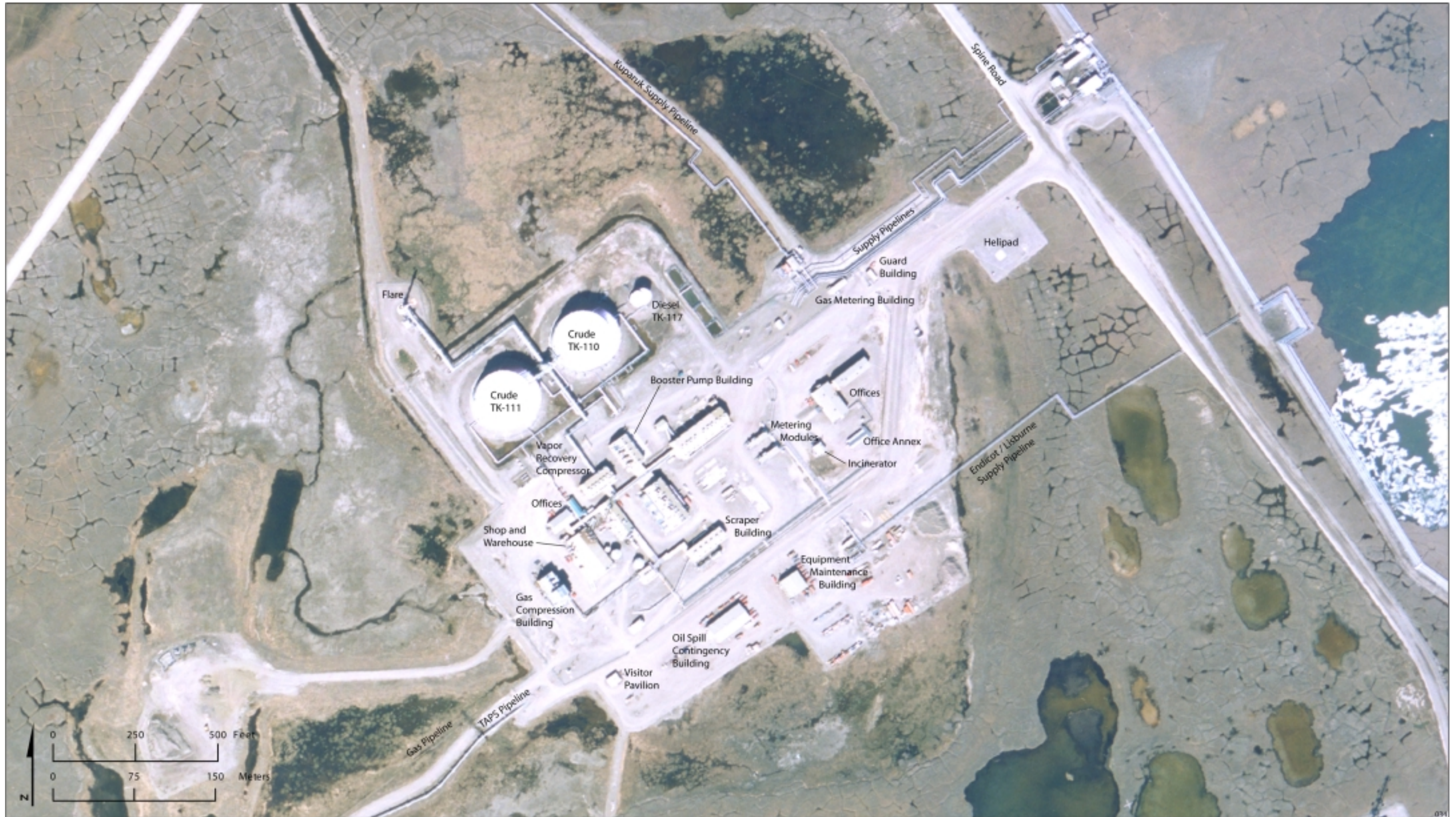
FIGURE 1-4 Example of a TAPS Pump Station
