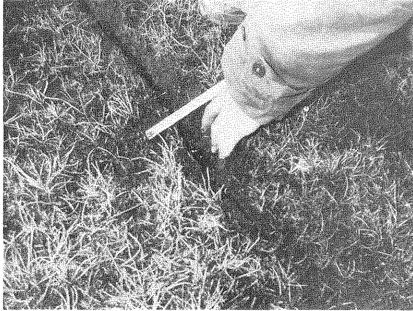
Fig. 2. This photograph illustrates the vertical tension crack in the tundra soils. This crack overlies a vertical wedge-shaped vein of ice.
