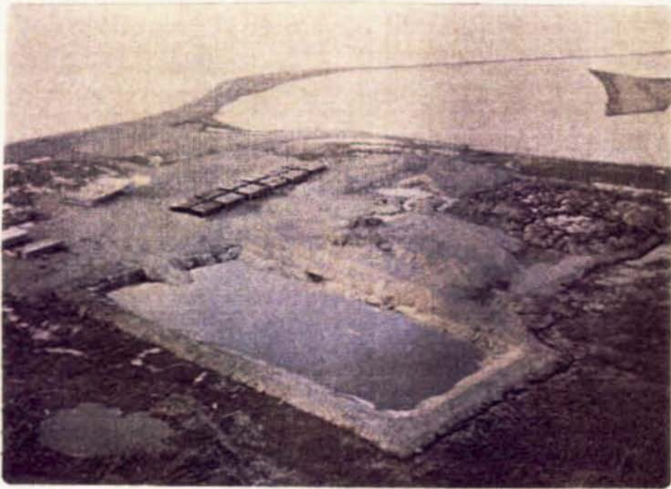
PHOTO 20. PT. THOMSON DRILLING PAD, MAINLAND SHORE
