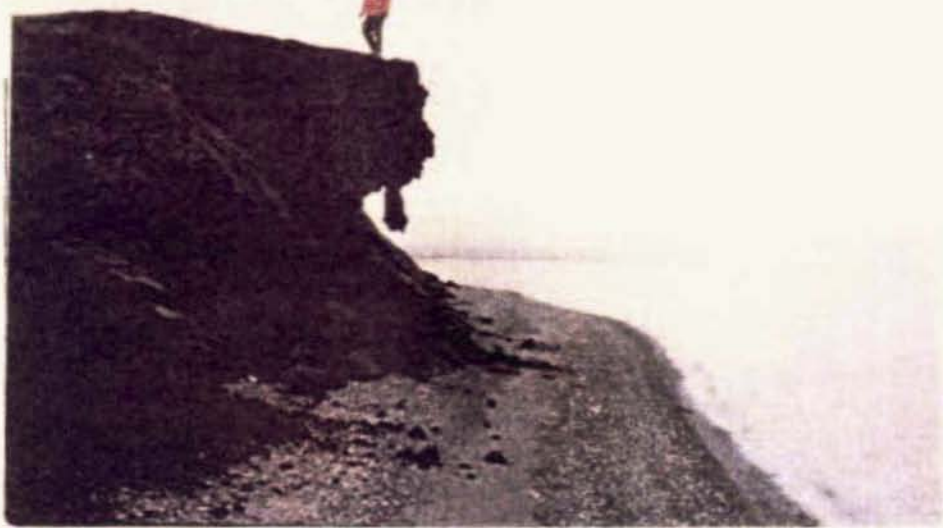
PHOTO 2. COASTAL BLUFF EROSION ON THE MAINLAND SHORE NEAR TRANSECT #5
