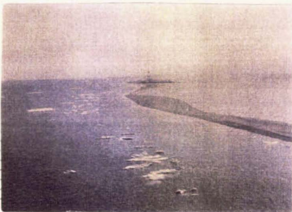
PHOTO 19. VIEW OF FILLED INLET THAT NOW CONNECTS DUCHESS AND NORTH STAR ISLANDS, JULY, 1982. EXXON'S NORTH STAR DRILLING PAD IS SEEN IN THE BACKGROUND
