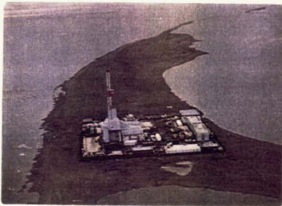
PHOTO 23. AERIAL VIEW OF THE NORTH STAR DRILLING PAD
