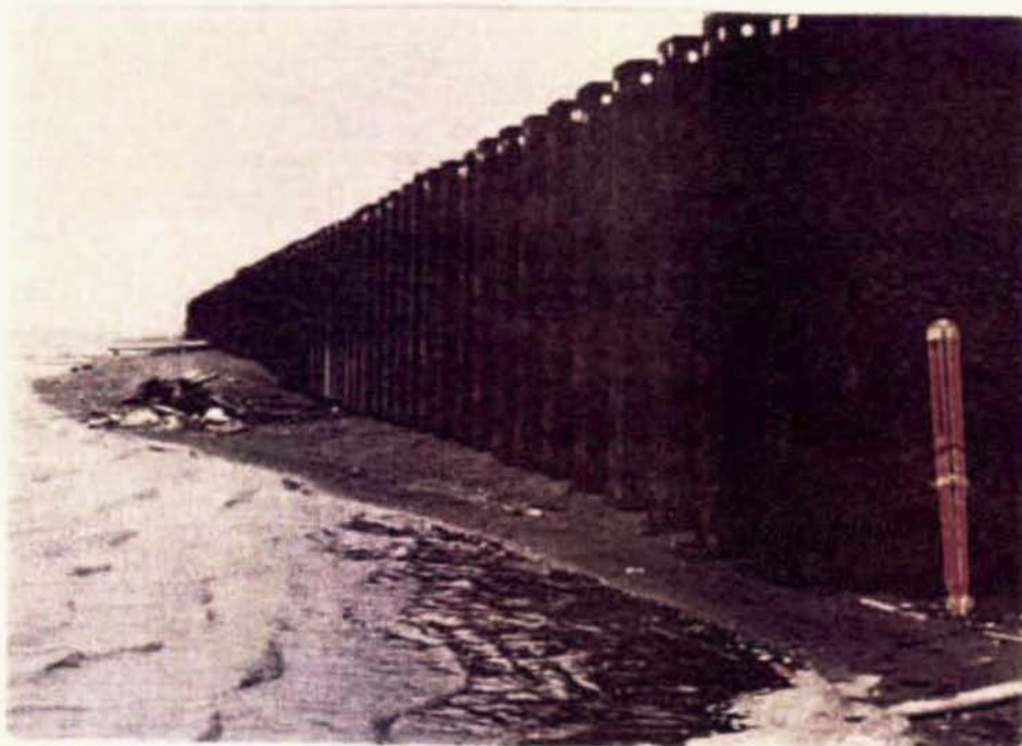
PHOTO 22. SHEET PILE WALL ON THE NORTH SIDE OF FLAXMAN ISLAND DRILLING PAD SHOWING THE CLOSE PROXIMITY OF THE WATERLINE
