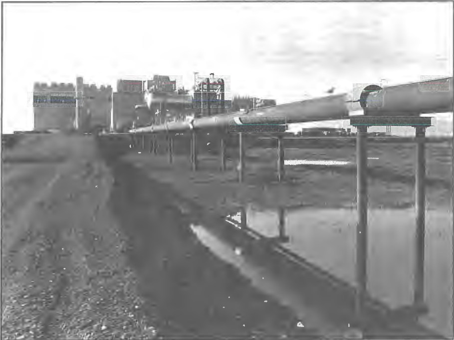
A North Slope pump station feeds the Trans Alaska Pipeline. (Photo courtesy of ARCO Alaska.)
