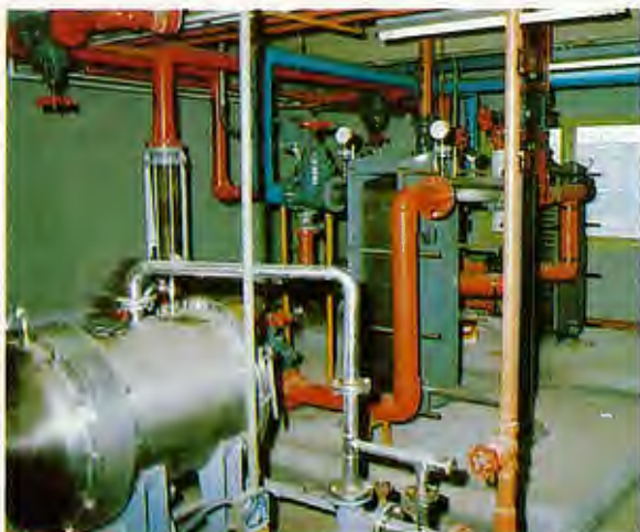
Heat exchanger used at a geothermal warm water abalone hatchery in Hokkaido, Japan. The warm water increases the growth rate of cultured abalone.
