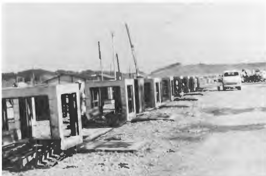
Figure 1.—Japanese concrete cube reef units (sides = 2 m) being built in Chiba Prefecture, Japan.
