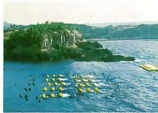
Floating breakwater used to develop a culture area in the outfall of a nuclear power plant in southern Japan.
