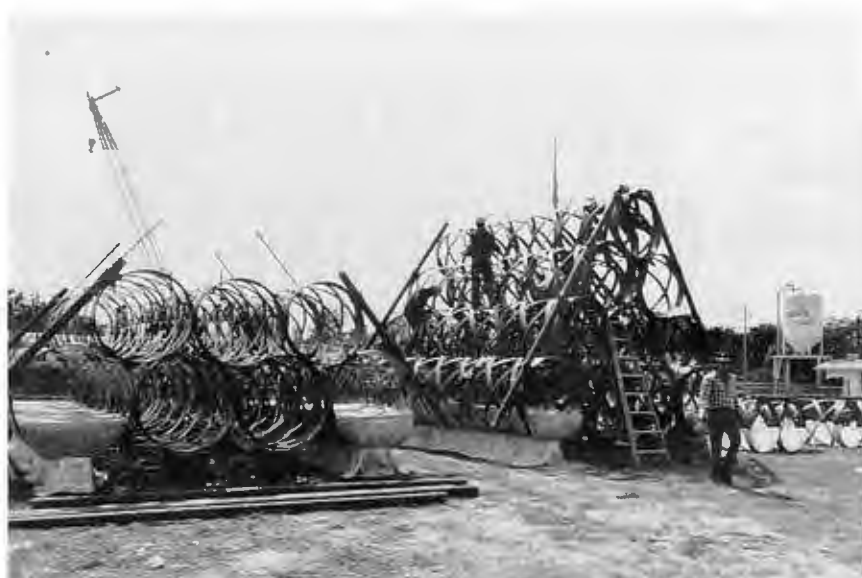
Figure 12.—Three types of FRP units built in Jacksonville, Fla. Concrete ballast has been placed in lower cylinders of largest unit.
