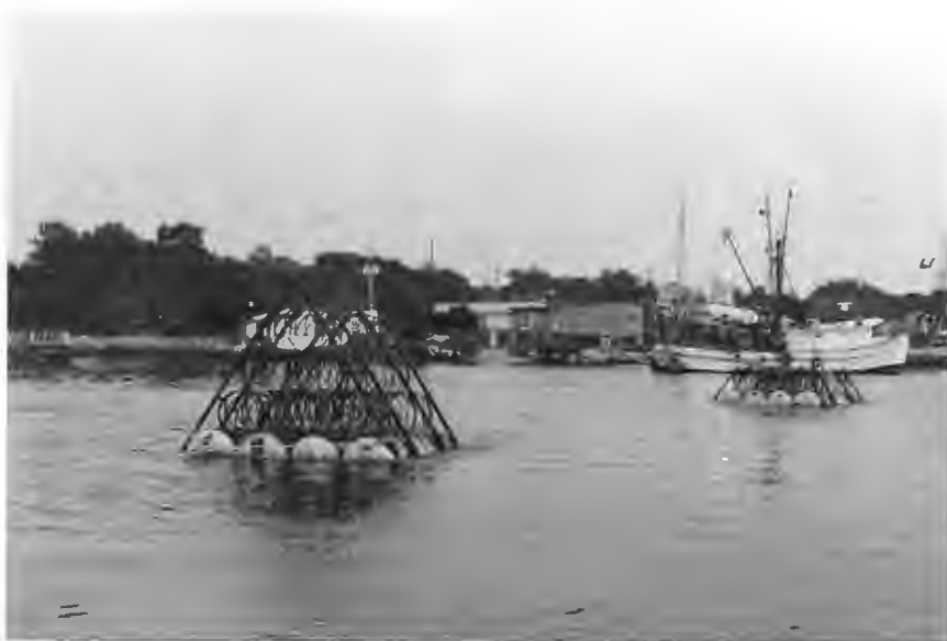
Figure 16.—Reef units being towed to site off Jacksonville, Fla.
