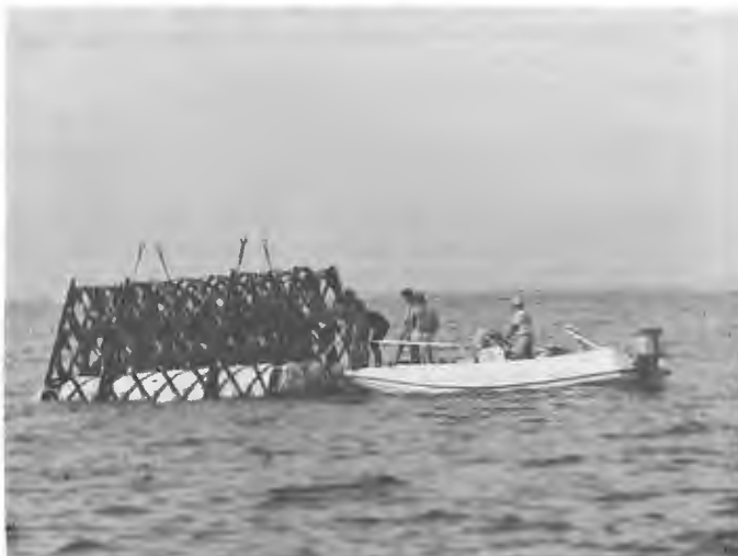
Figure 2. FRP Unit with Airbag Flotation System Maneuvered into Final Position off Panama City, Florida.
