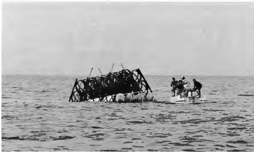
Figure 17.—Reef unit being sunk on site off Jacksonville, Fla.
