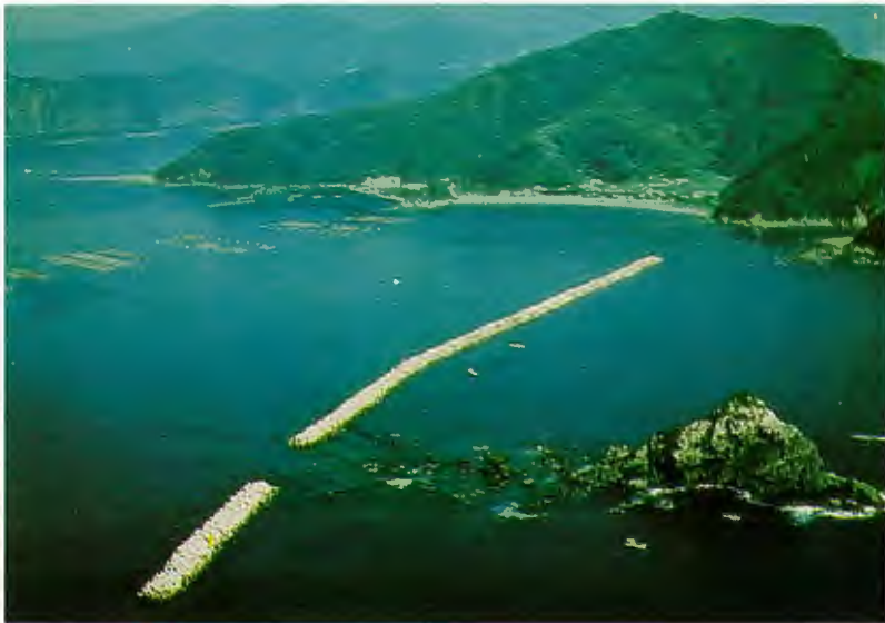
Large tetrapod breakwater used to create sheltered culture areas. (Photo courtesy of Nippon Tetrapod Co., Ltd.)
