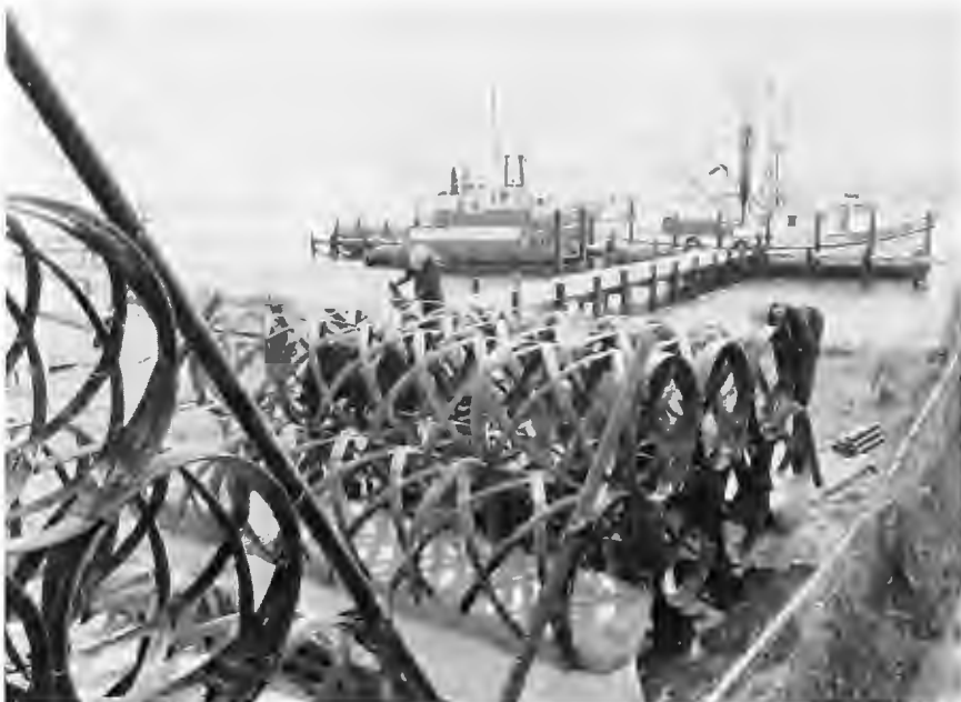
Figure 14.—Workers fibreglassing all connecting points.
