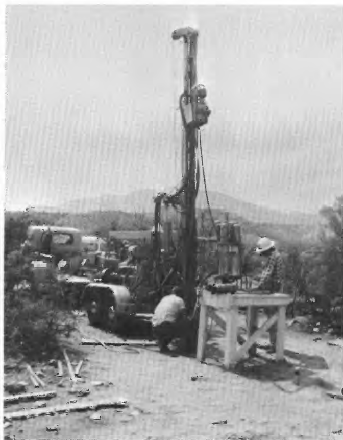
FIGURE 8.—Hydraulic rotary vacuum drill used to install soil-moisture wells.
