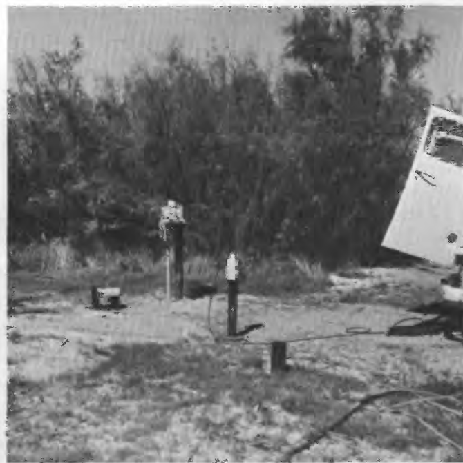
FIGURE 9.—Typical observation site, showing observation well with digital recorder and soil-moisture well with neutron-moisture meter in place.
