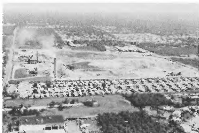
FIGURE 7.—View of Islip landfill, looking north. Incinerator facility is at center left with large smokestack. Old incinerator beyond it (to north) has stack without smoke. Sand and gravel is not currently (1974) mined here, but a gravel-washing operation is at lower right of landfill. Water-table ponds are in right center. Photograph taken June 13, 1974.
