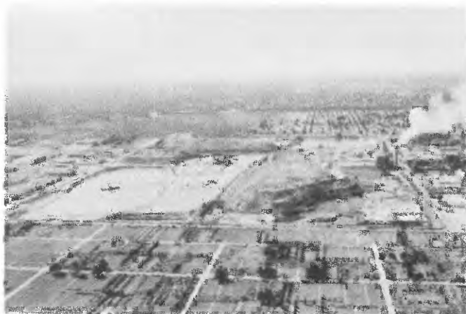
FIGURE 6.—View of Babylon landfill, looking south. Incinerator facility is at right. Sand-and-gravel operation, center left, is in water-table pond. Scavenger-waste-facility ponds are to the front and right (north and west) of large refuse pile in center. Photograph taken June 13, 1974.
