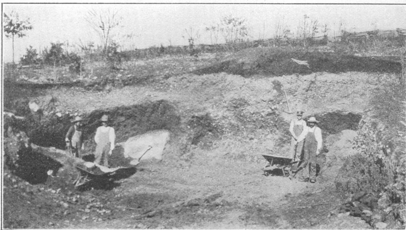
C. HAND MINING BY PICK AND SHOVEL IN OPEN CUT AT CUTTER MINE.
