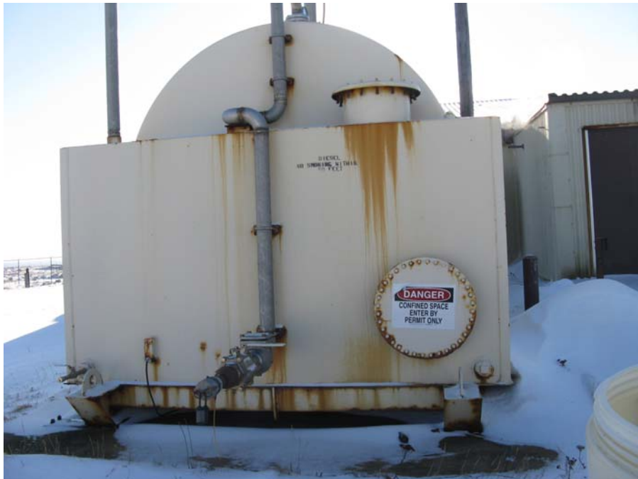
Photo No. 10 Building 110 AST
