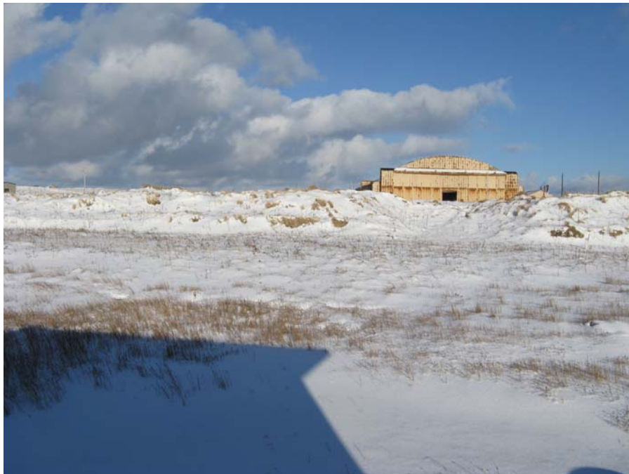
Photo No. 4 Water Gallery View Looking North
