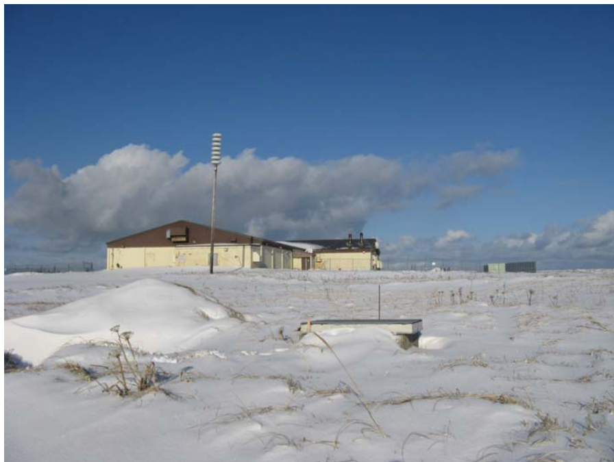
Photo No.14 Building 110
