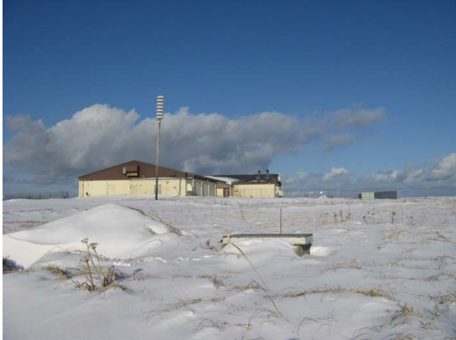
Photo No. 9 Building 110 Looking North
