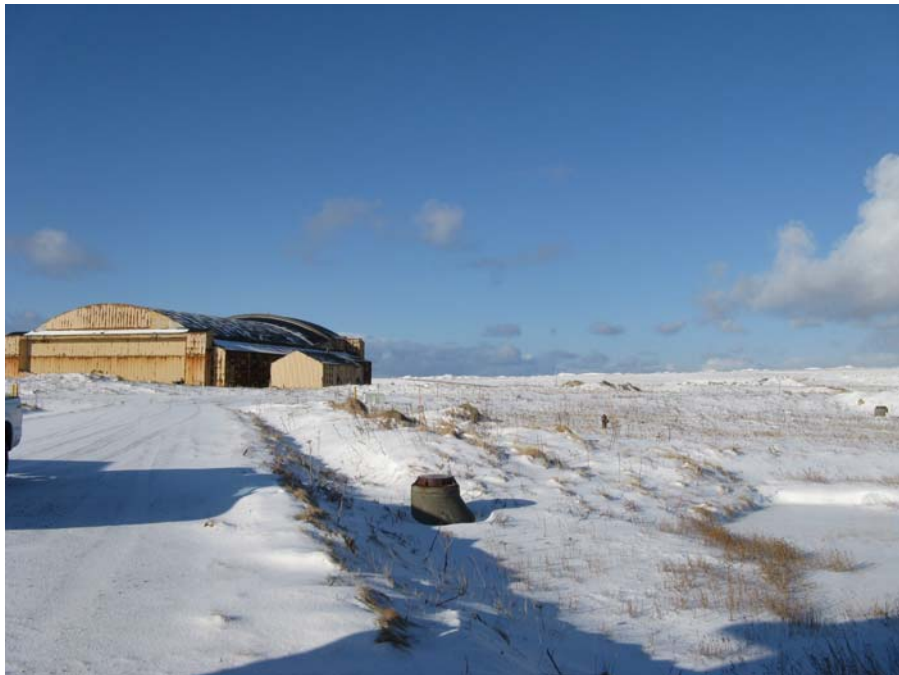
Photo No. 2 View Looking West, Building 705 – Water Gallery
