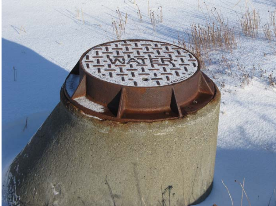
Photo No. 1 Water Gallery Access
