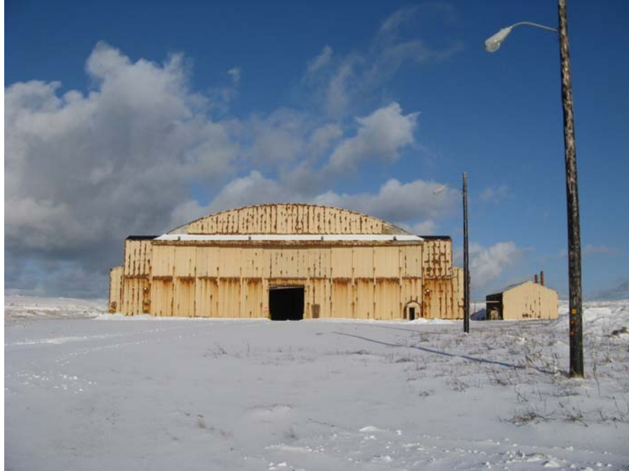
Photo No. 13 Hangar 4
