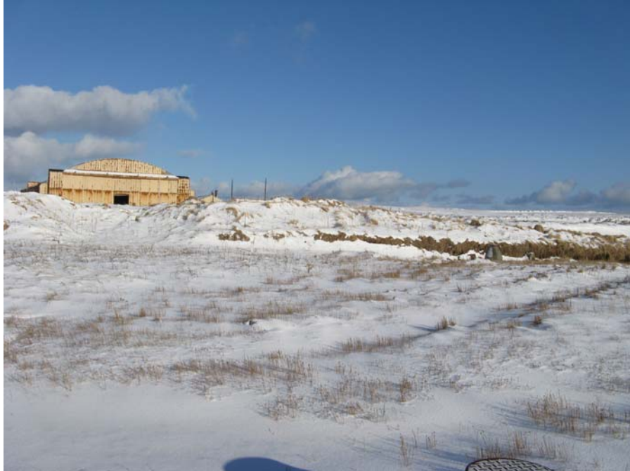
Photo No. 5 Water Gallery View Looking Northeast
