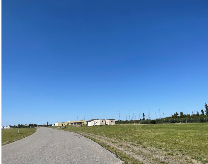
Photo No. 1 WL0B1 and WTP Looking West
