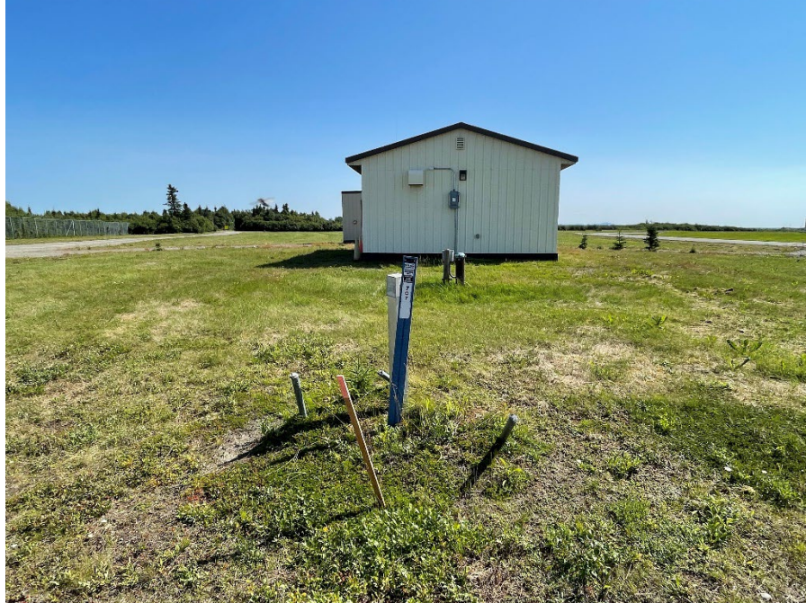
Photo No. 5 Monitoring Well 707 in front of WL0B1 and WTP View Looking East
