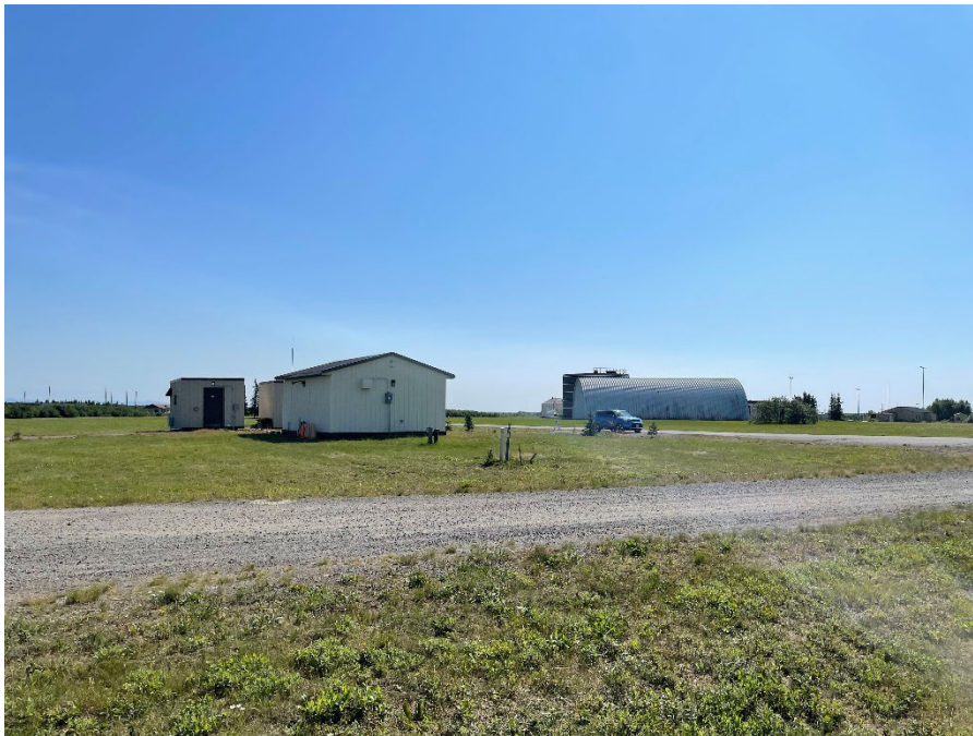
Photo No. 2 WL0B1 and WTP Looking East
