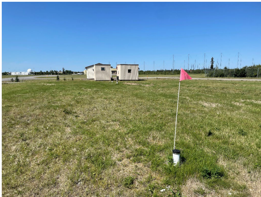
Photo No. 4 Soil Absorption System near WTP for the GAC & Microlite Filter Backwash View Looking Northwest
