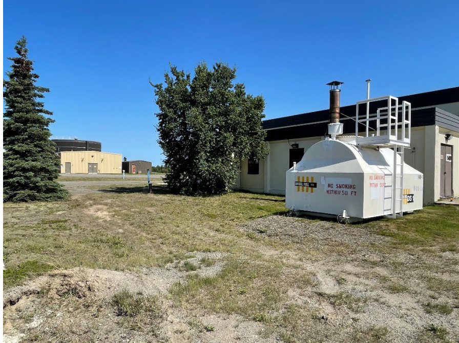
Photo No. 7 Typical Building Double Walled Fuel Tank – Outside of Source Protection Area View Looking Northeast
