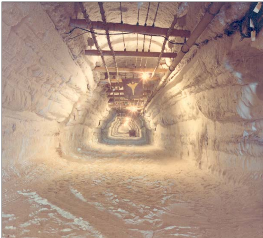
Figure 16. Main 400-m-long access trench below the surface at Camp Century, 1964. More than a dozen, 150-m-long side trenches radiated out from the main trench.
