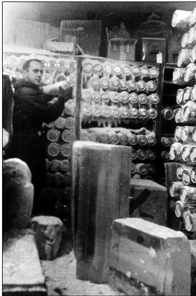
Figure 20. One of the ice core storage freezer compartments at CRREL, 1965.
