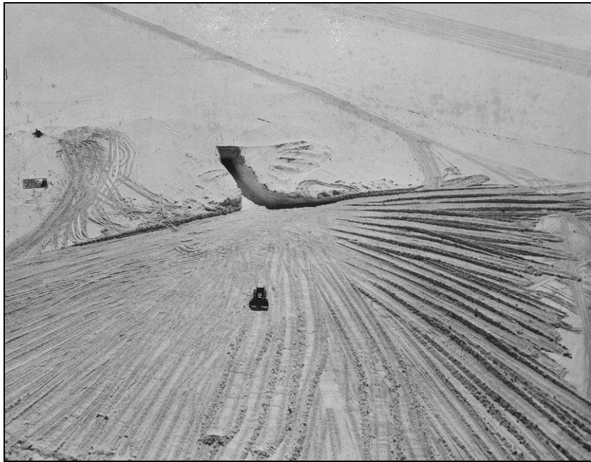
Figure 15. Surface view of the ramp entering below surface Camp Century complex, 1964. The D9 Caterpillar tractor is clearing snowfall and drift to allow easy access to the entrance.
