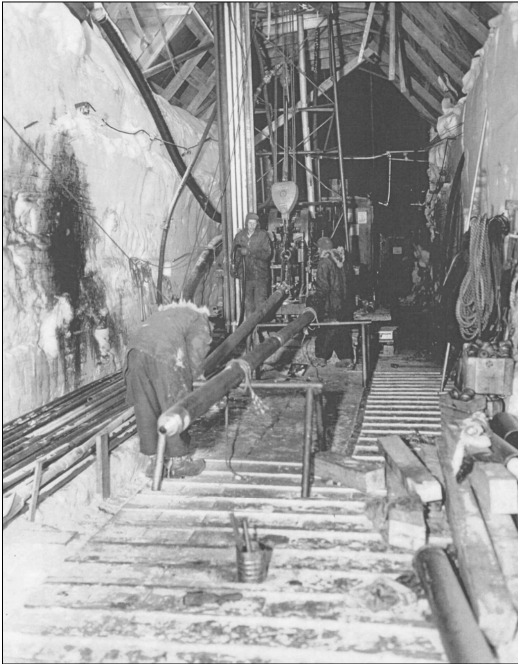
Figure 8. Below-surface core drilling trench with crew at the rig's borehole, 1957.
