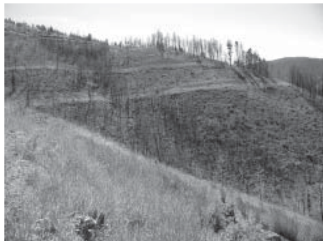
Figure 4 —Jammer road rehabilitation, Bitterroot NF (photo by Craig Odegard).
