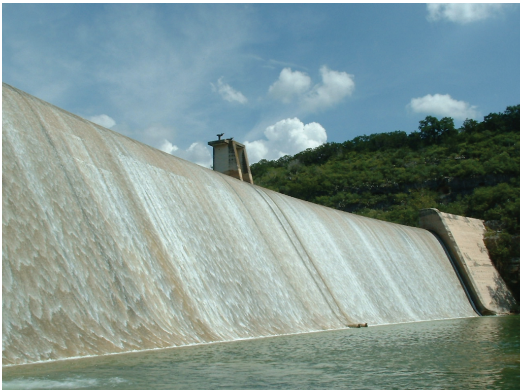
Figure 6. Diversion Dam near Riomedina, Texas, August 2004.
