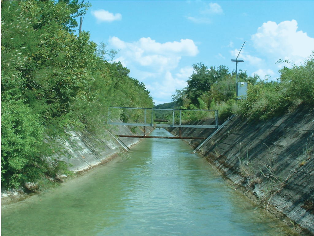
Figure 5. Medina Irrigation Canal near Riomedina, Texas, August 2004.
